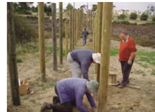
Volunteers constructing boardwalk
