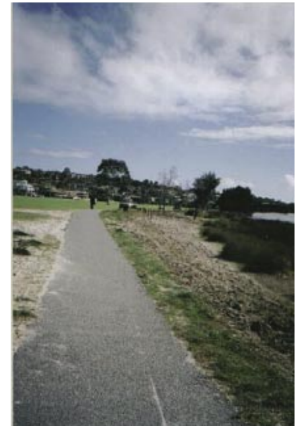
Area to be fenced along Attadale foreshore separating pedestrians and dogs from shorebird habitat.
